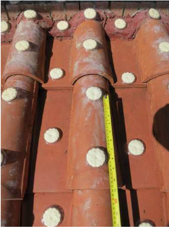
Figure 4. South roof treated with Bird Free .
