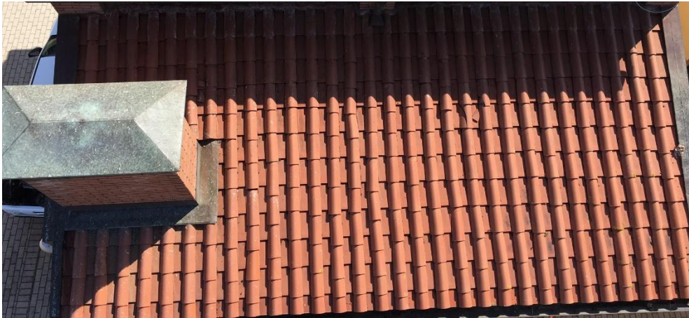
Figure 8. North roof after cleaning.
