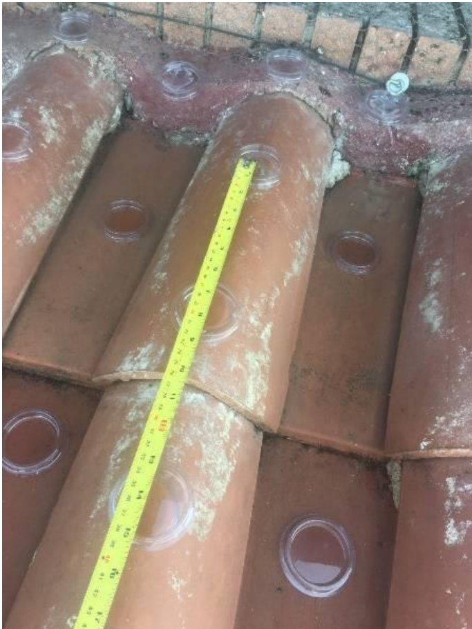
Figure 9. North roof treated with empty PET dishes as a “control”.
