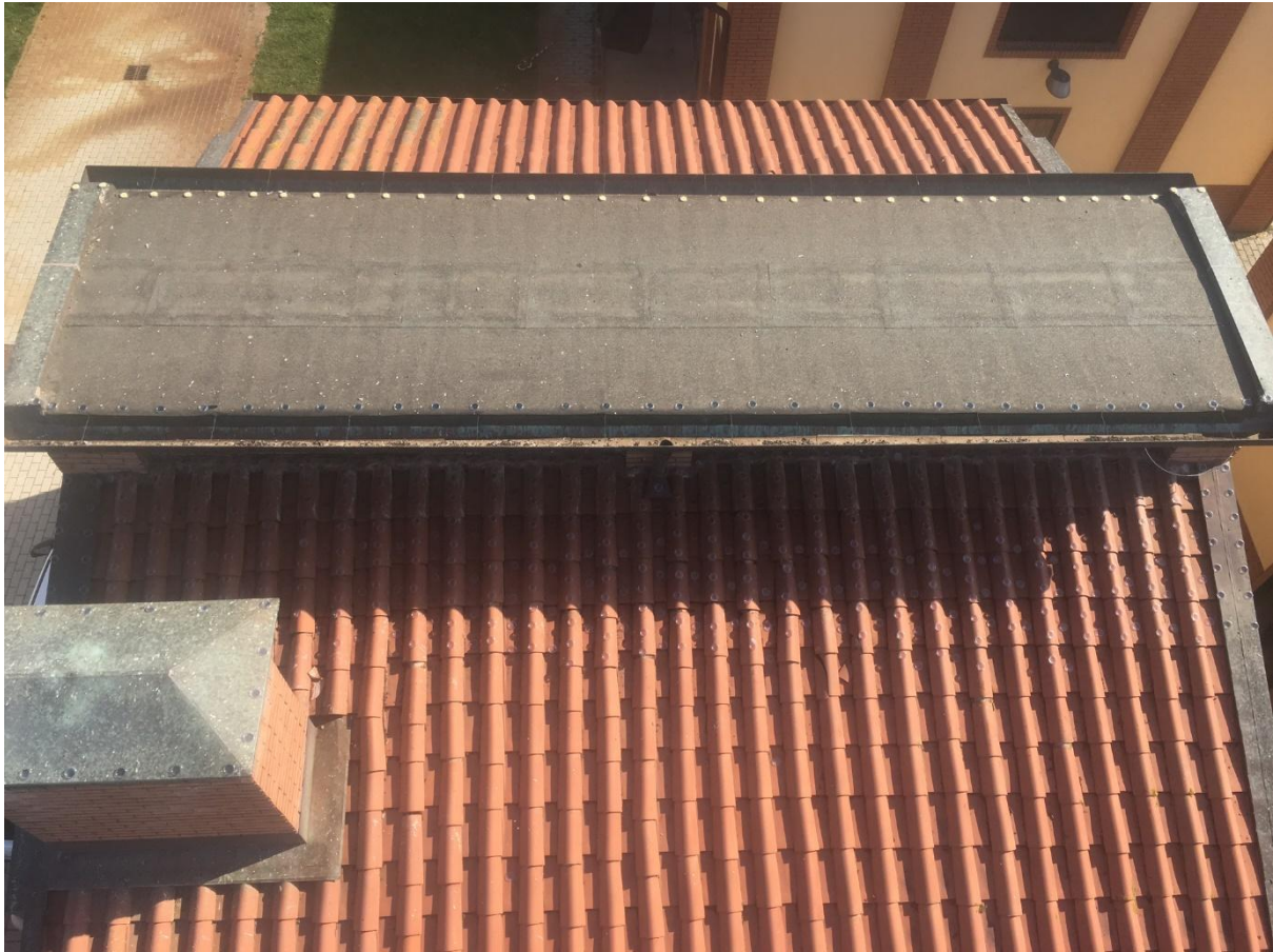
Figure 10. The area of the north roof treated with empty dishes was approximately 9m x 1.8m.
