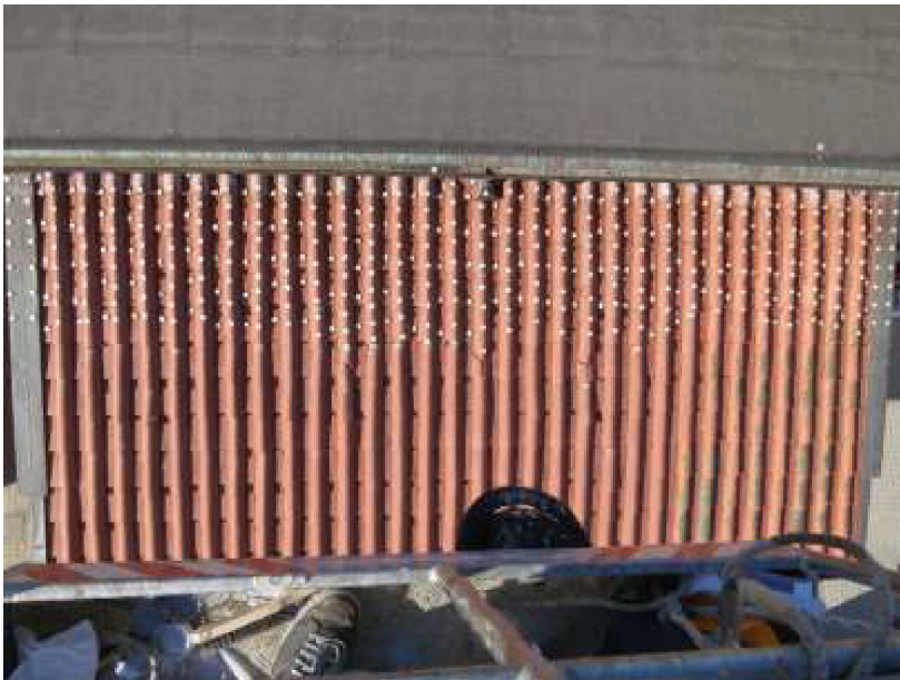
Figure 5. The area of the south roof treated with Bird Free was approximately 9m x 1.8m.
