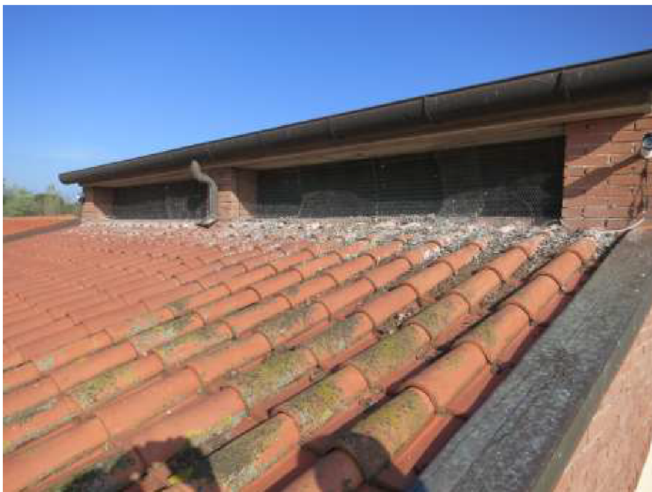
Figure 1. South roof prior to cleaning and treatment.
